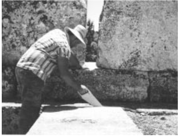
Fig. 14. Sawing a joint.
