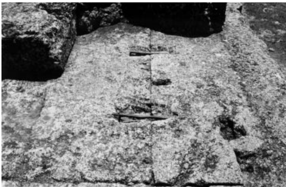
Fig. 12. Two ancient iron clamps partially pulled from their blocks.
