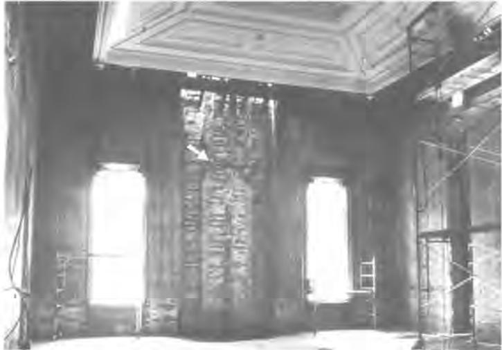
South Hall. University of California, Berkeley. During retrofit in the 1980s. Wall coverings and fireplace flue bricks have been removed. Horizontal pieces of bond iron can be seen running across the flue between tops and sills of the right and left windows.
