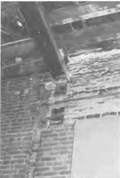
South Hall. University of California, Berkeley. During retrofit in the 1980s. Edge of vertical iron T column and iron girders exposed after wall excavation. Bond iron can also be seen in front of the T column. *Photograph by author.*
