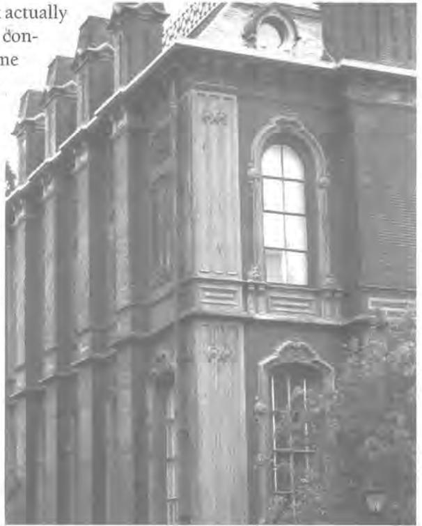
South Hall. University of California, Berkeley. Southeast corner illustrating pilasters which are fastened to bond iron and threaded rods by decorative nuts at the level of the window cornices on each floor.
