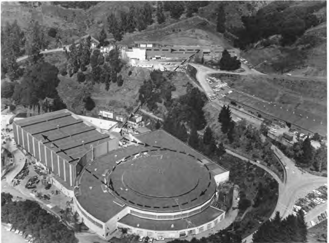
Exterior view of Bevalac: arrows show path of particles from SuperHILAC at top, down the transfer line to Bevatron at bottom, finally to target areas within High-bay Building next to Bevatron, April 1975. LBL Photographic Services CBB 766-4673.
