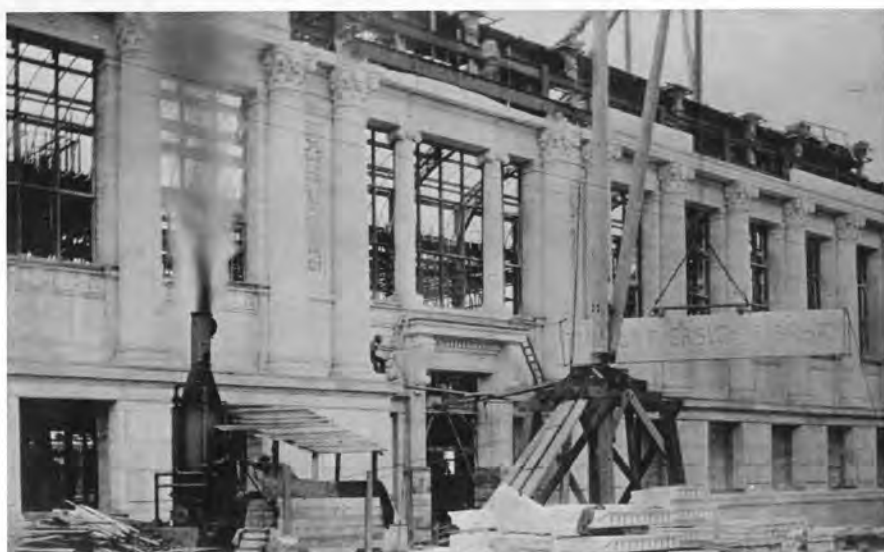
Construction of north façade of Doe Library, with University Library block being lifted into place above main entrance, 1909. University Archives (UARC PIC 9:24).
