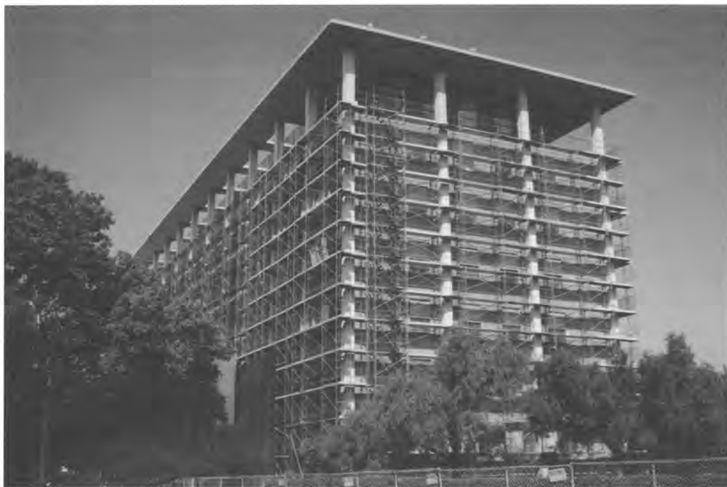
Seismic retrofit of Barrows Hall, 2000. Photograph by Catherine Dinnean.
