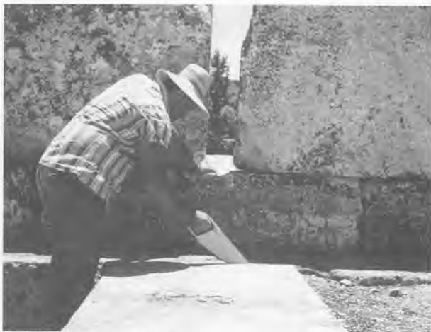
Fig. 14. Sawing a joint.
