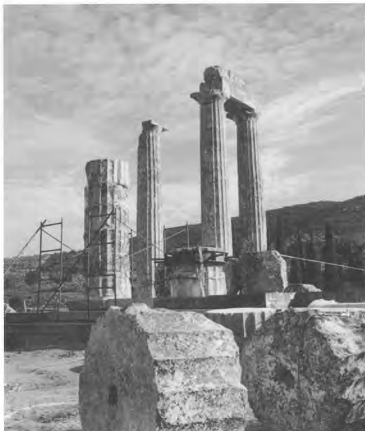
Fig. 16. Two “new” columns going back in place (six drums set on one, two on other, of total 13 in each) on November 29, 1999.
